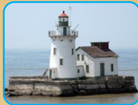
Cleveland West Pier
